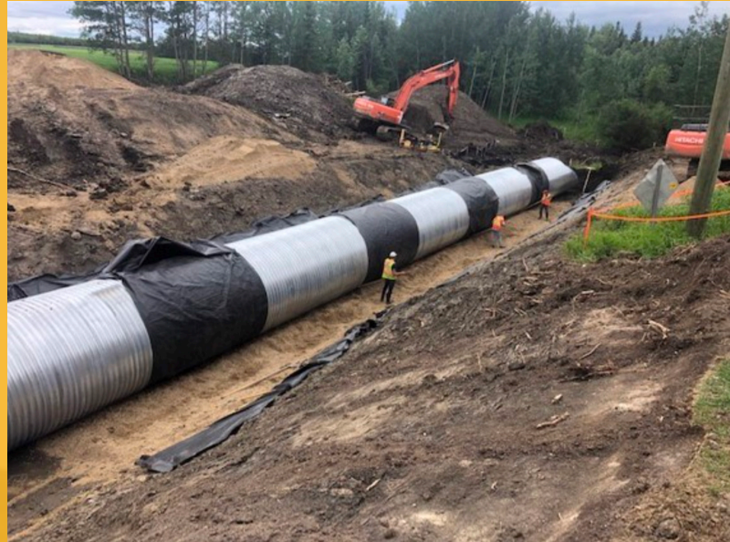
Range Road 104 Culvert Replacement - Completed July 2019 Location: NW 4-79-10-W6
