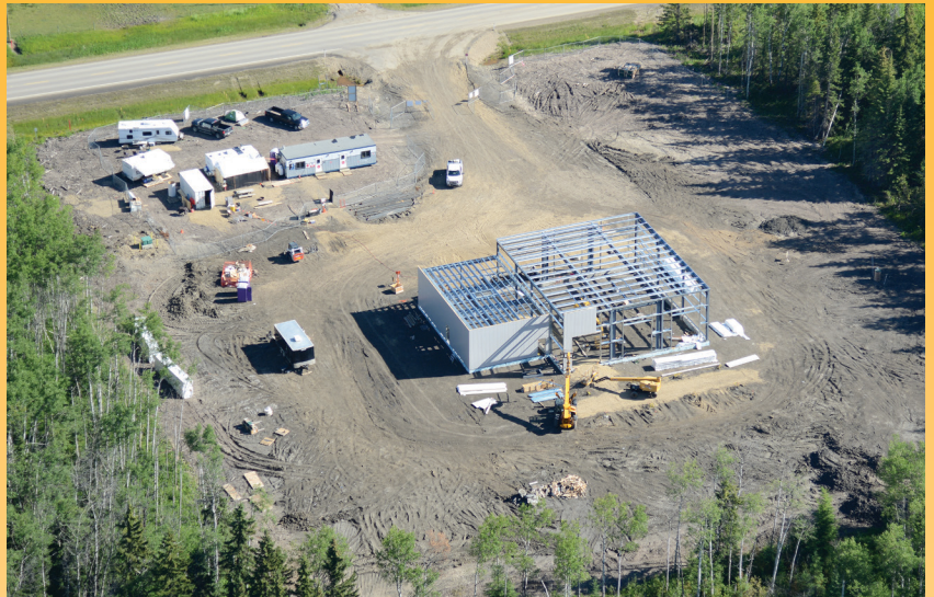
Aerial view of new Savanna fire hall
