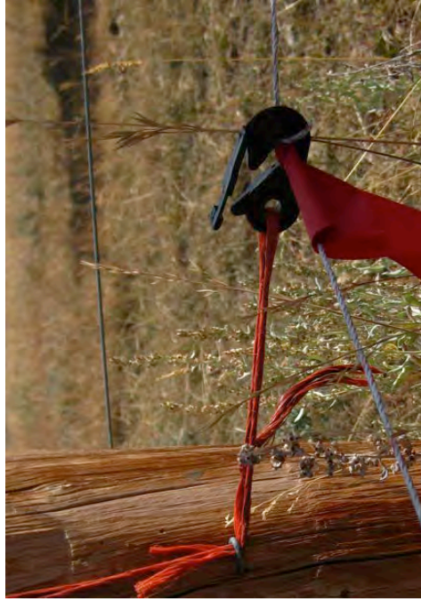
Figure 8: Tensioning anchor, using a Dare brand insulated clip and twine to connect the fladry line to a permanent post.
